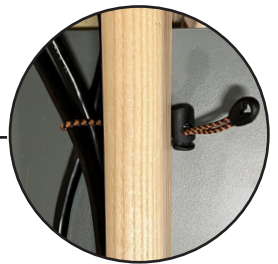
These bungee cords can be used to manage cables under the surface.
